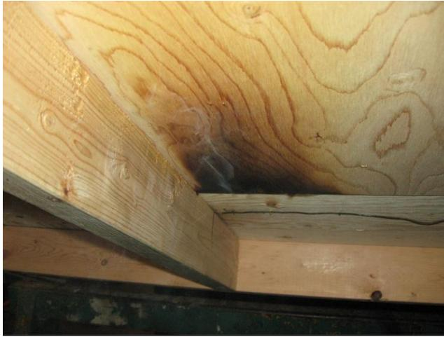
**Figure 30 - Unexposed Surface of Combustible Deck**
