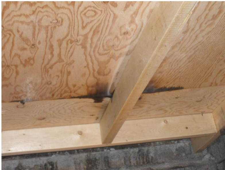
Figure 34 Photograph of Burning Brand on Module for Class A Shingle Roof with Class C PV and 0” Gap
