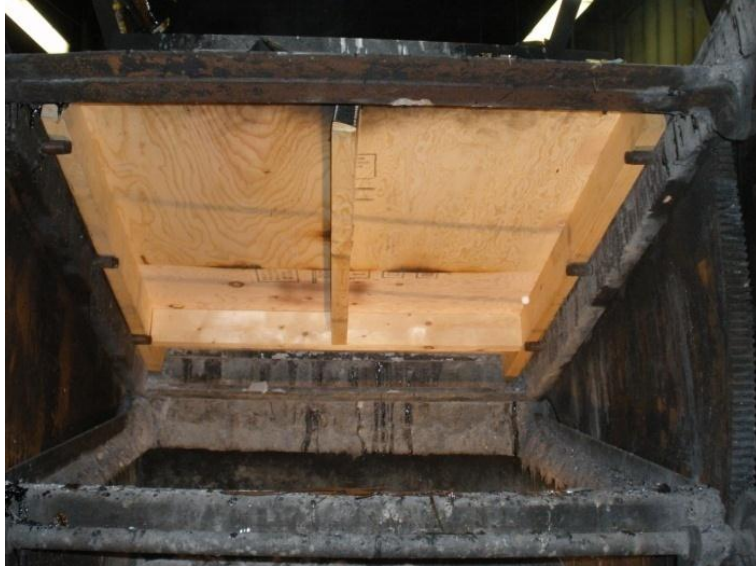
Figure 49 Underside of Roof Deck View: Burning Brand Test for Class A Shingle (3 tab) roof with Class C PV where Class A brand was located on the surface of the roof under the module
